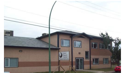
The new building in Regina
